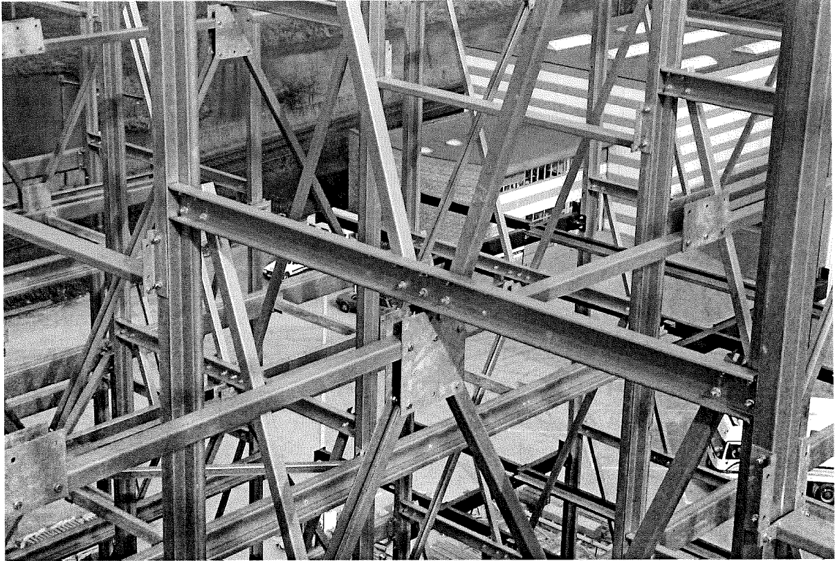
Fig. 2.12. Down-aisle bracing system
