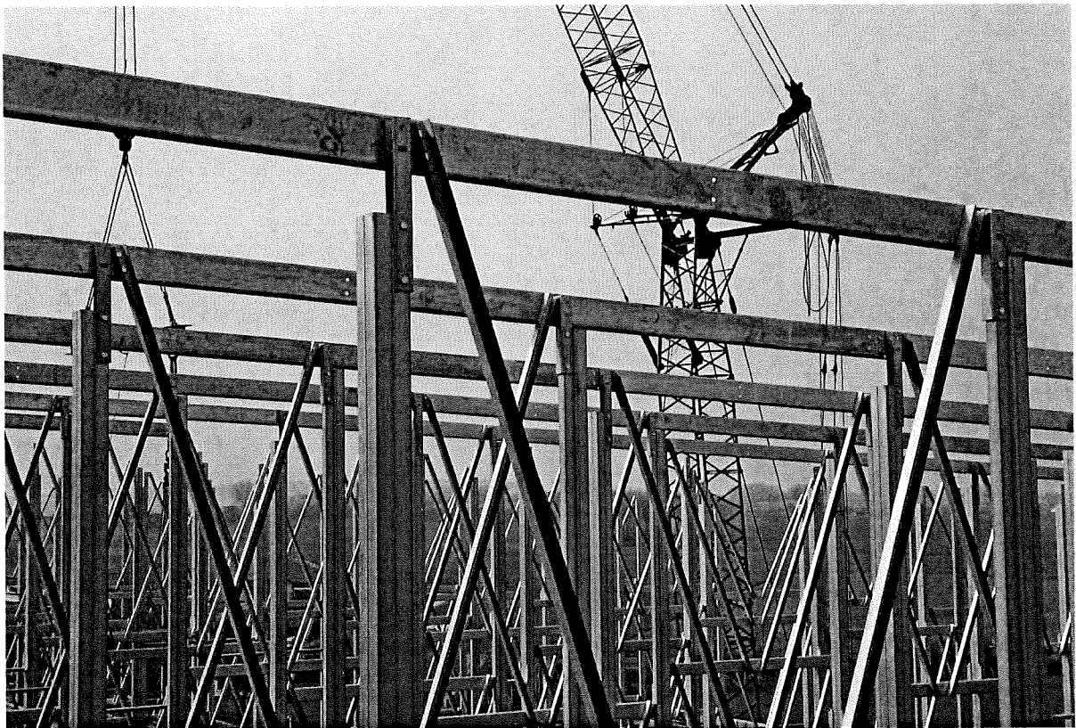
Fig. 2.12. Down-aisle bracing system
