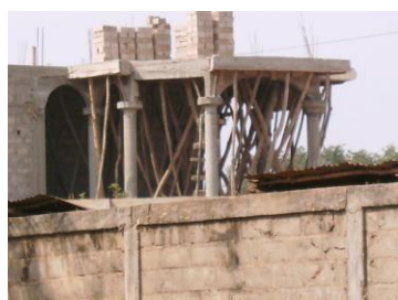
c: Stake for building suspended slab.
