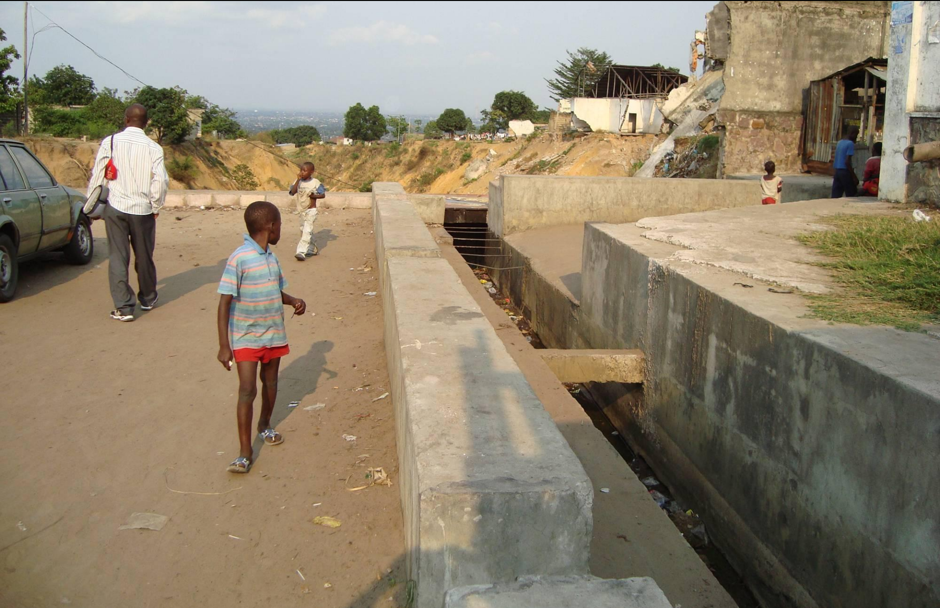
Canalisation of runoff
