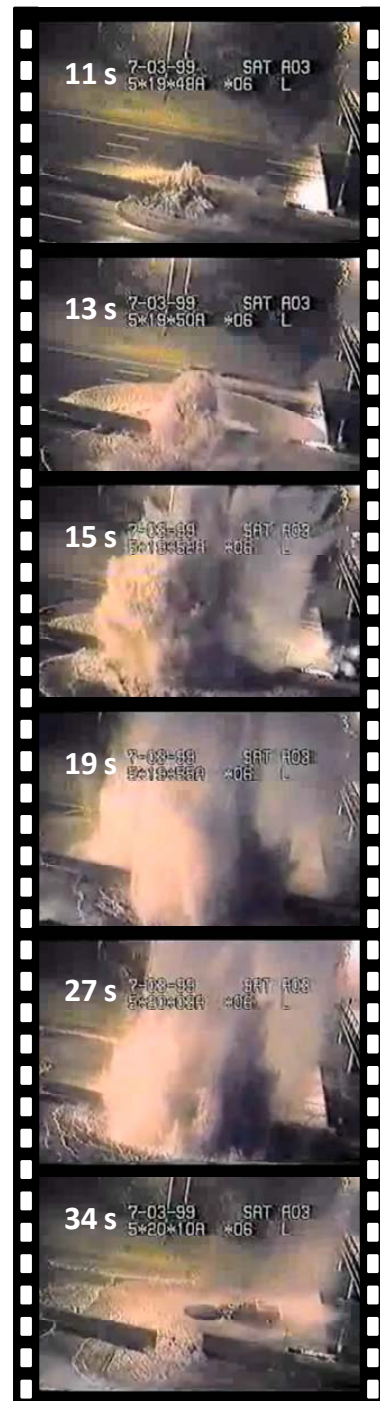
Figure 14: Storm-water storage tunnel - Chicago TARP
