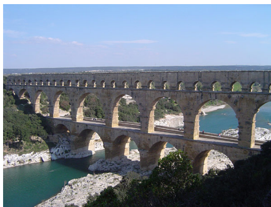
Figure 21: "Pont du Gard" is one of the most famous hydraulic structures from the ancient era.
