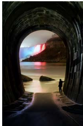
Figure 12: Tailrace tunnel of the Rankine Generating Station in Niagara Falls [149]
