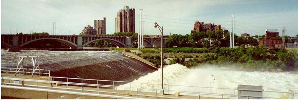
Figure 7: Saint Anthony Falls on the Mississippi River shows a pronounced Hydraulic jump
