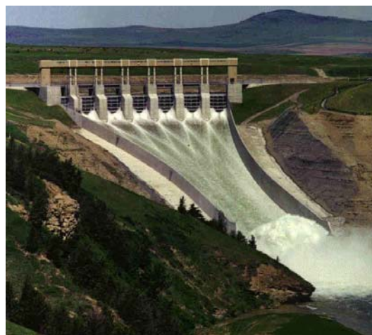
Figure 6: Spillway of the Oldman Dam (USA) [2] - air entrainment on side walls is created by the intersection of the free surface with the side-walls boundary layers
