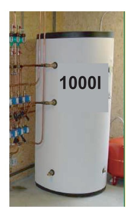
Solar collector field feeds a hot water storage. If it reaches 65°C (minimal temperature for the chiller operation), a certain amount of heat
