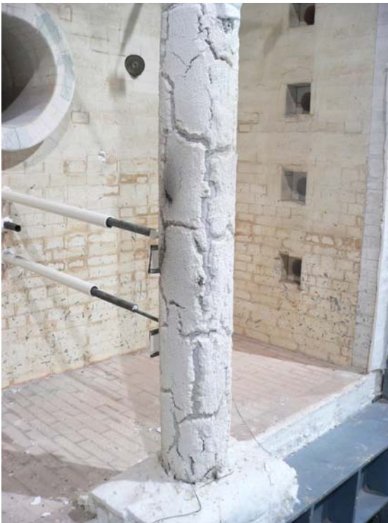
Fig. 5 Intumescent paint of column 4A after the test
