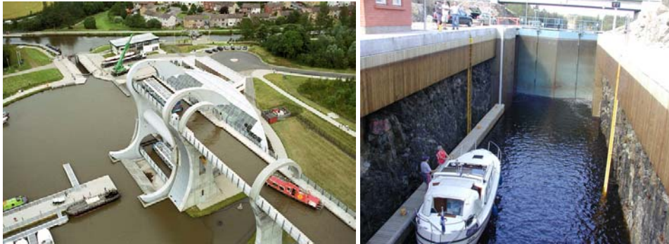
Figure 6. Project reviews: Falkirk Wheel - UK (left), Floating Pontoon and lock in the rock – Finland (right)
