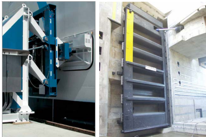
Figure 5. Examples of Project reviews – Mooring System (Left), Folded plate miter gate and capsulated hydraulic actuator (right)
