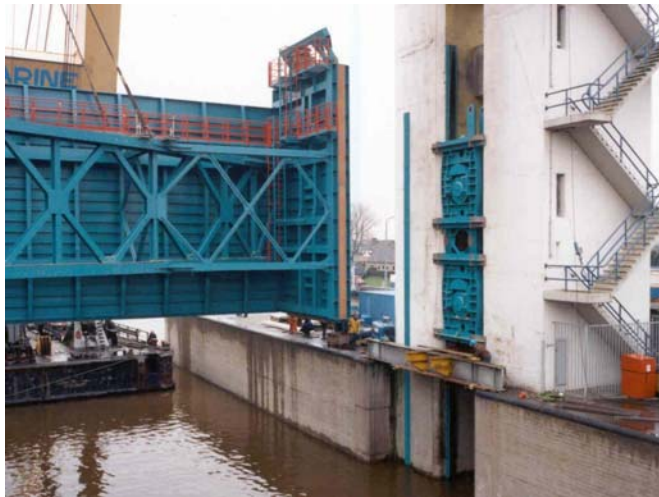
Figure 14. Vertical lift gate guides in Krimpen a/d IJssel (left) and in Hartel Canaal Barrier (right)
