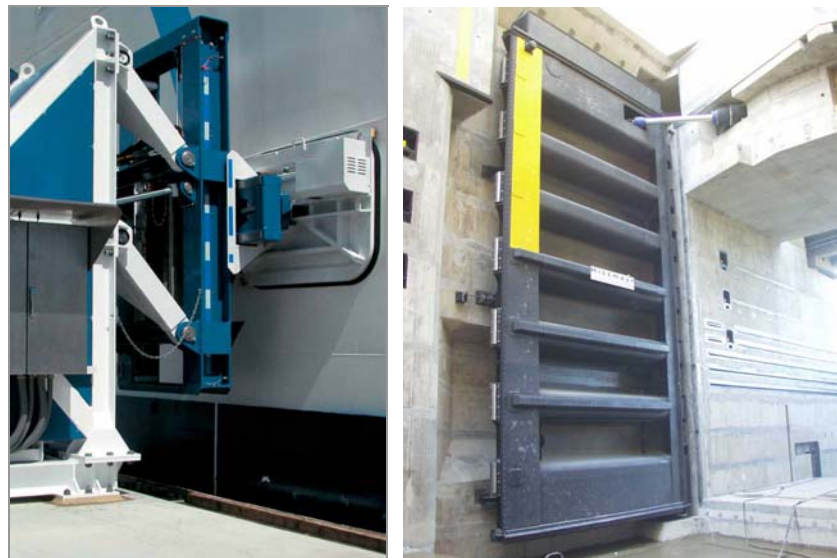
Figure 6: Examples of Project reviews – Mooring System (Left), Folded plate miter gate and capsulated hydraulic actuator (right)
