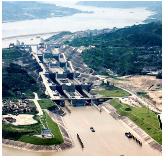
Figure 8: The Three Gorges Project (China)
