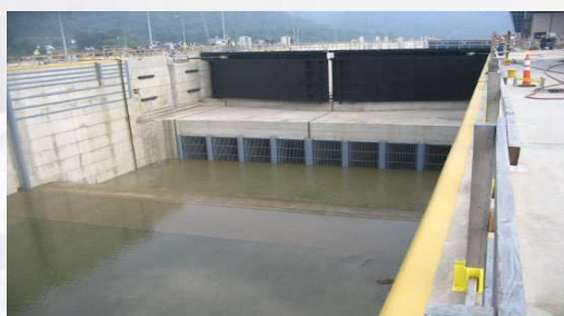
In Chamber Longitudinal Culvert System (ILCS) (Fig. 4.16)
