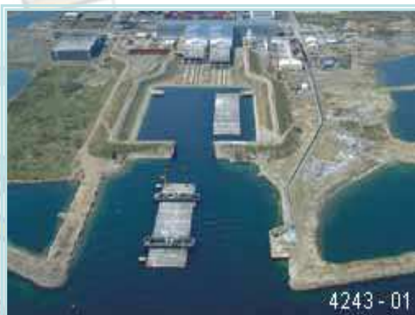
Immersed tube tunnels (Float-In)
