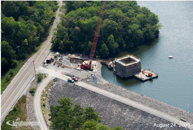
Precast Lock Segments on Barges
