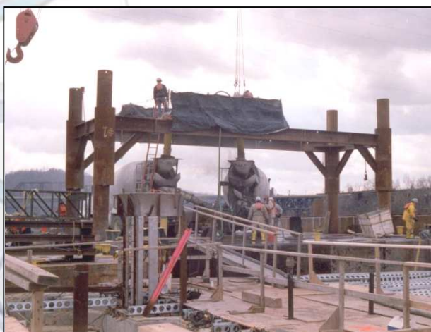
Grouting the Foundation 2000 m3 Of Underbase Grout under Water
