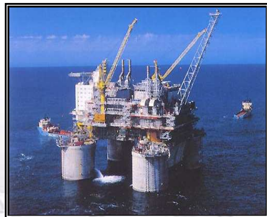
Offshore drilling platforms (Float-In)
