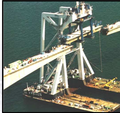
Float-in Construction of Tacoma-Narrows Bridge Pier
