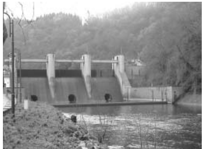
Figure 9 Downstream view of the Nisramont dam (© HACH).
