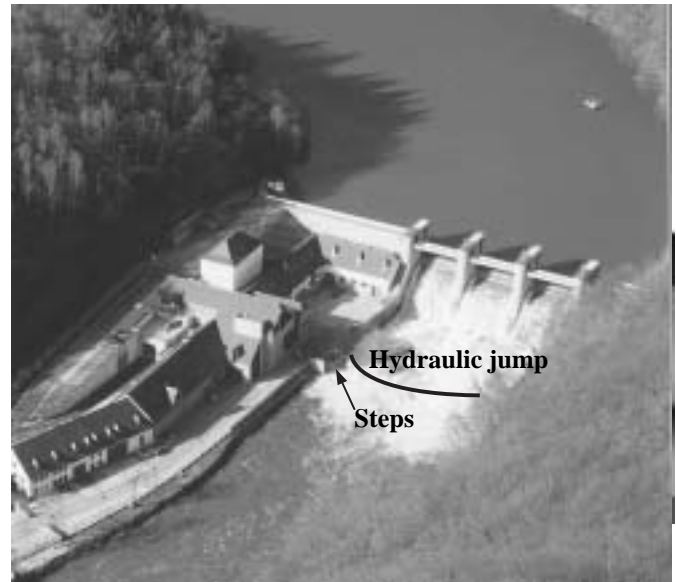
Figure 11 175 m 3 /s flood on the spillway (© MET).
