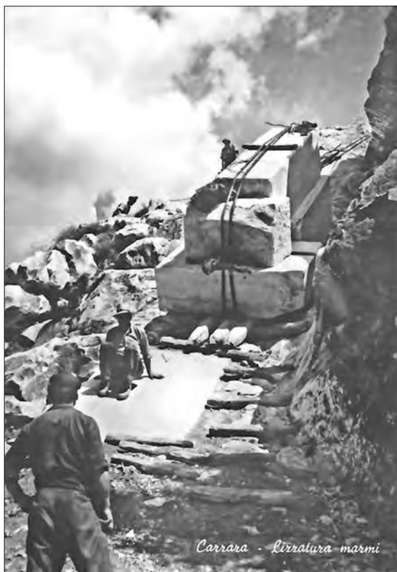
Fig. 12 - Lizzatura at the marble quarries of Carrara, Italy, early 1900's postcard.
