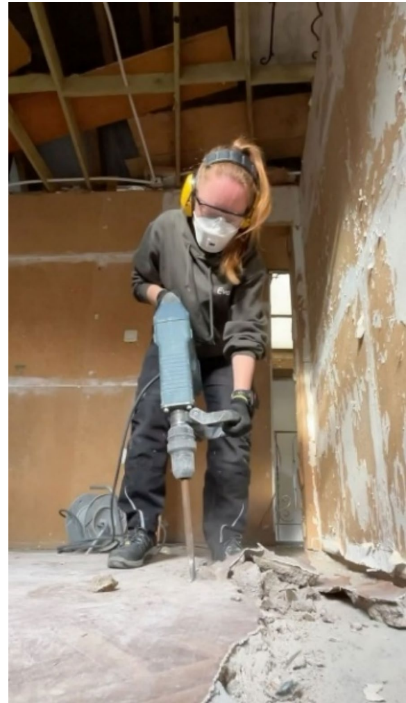
Fig. 13 ChatGPT Description of the photo: a woman is using a power tool (jackhammer) to break apart the floor inside a building. The background shows a construction or repair setting with exposed beams and walls
