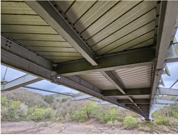
Figure 3.4: Underdeck, with its main components: cross beams and longitudinal beams.
