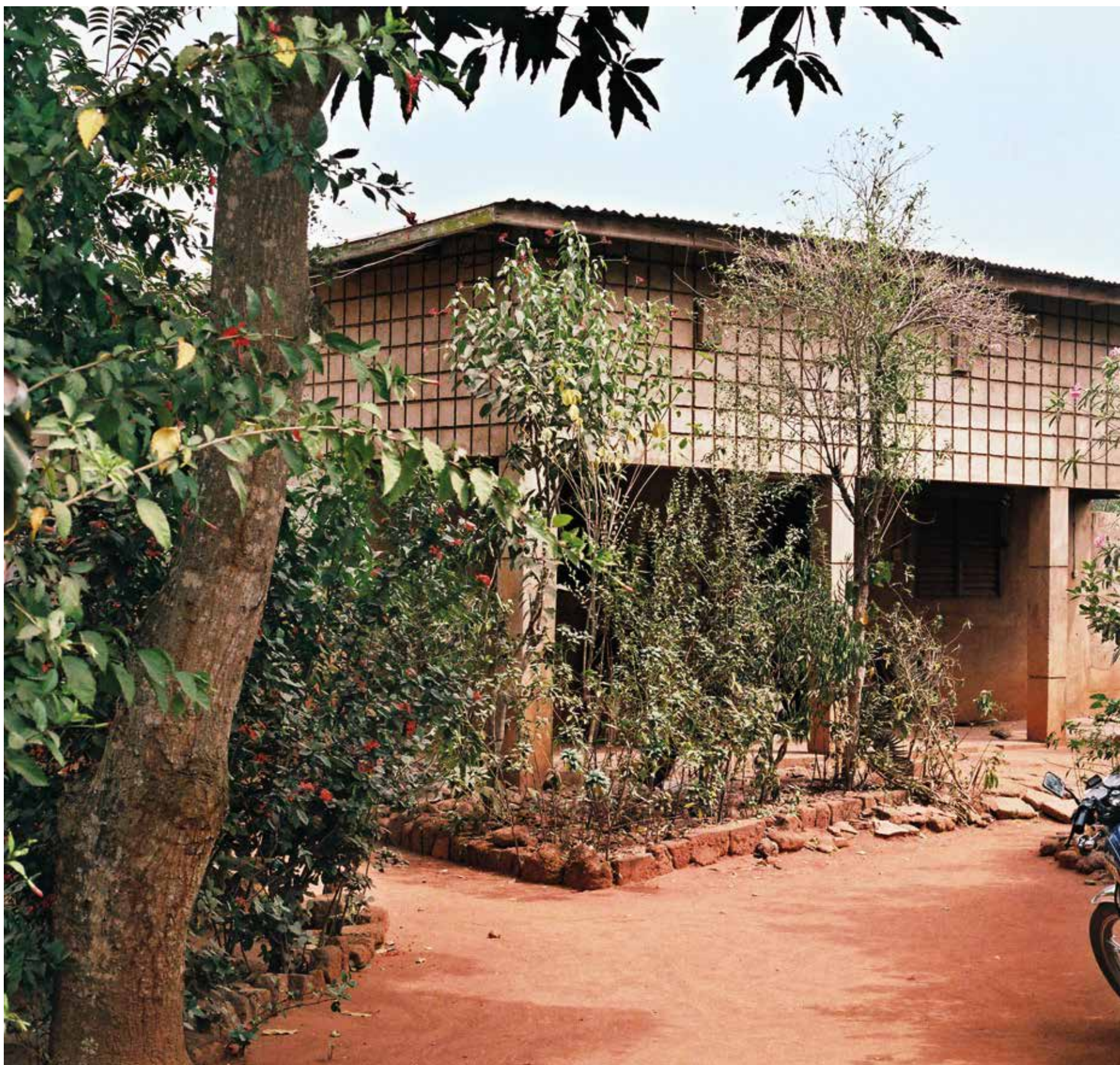
Courtyard of Bah Nondichao's house from the gate. Zongo neighbourhood, Abomey, 10 Jan 2015
