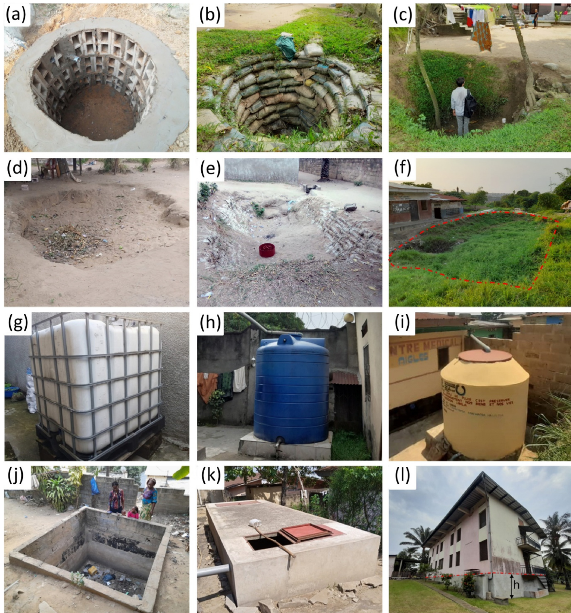
Fig. 3. Illustrations of observed runoff retention measures used to collect, store and infiltrate rainwater. (a) losing well with blocks; (b) infiltration pit with sand bags; (c) retention basin with vegetation; (d) poorly maintained retention basin filled with sand; (e) partially filled retention basin with sand bags; (f): vegetated retention basin allowing high infiltration rates and avoiding bottom clogging; (g) & (h) plastic rainwater tanks (small and large capacity); (i) cement rainwater tank; (j) open underground tank in masonry collecting rainwater from roofs; (k) closed underground tank in masonry; and l: cellar serving as tank collecting rainwater from the roofs, occupying the entire underground part of the building.
