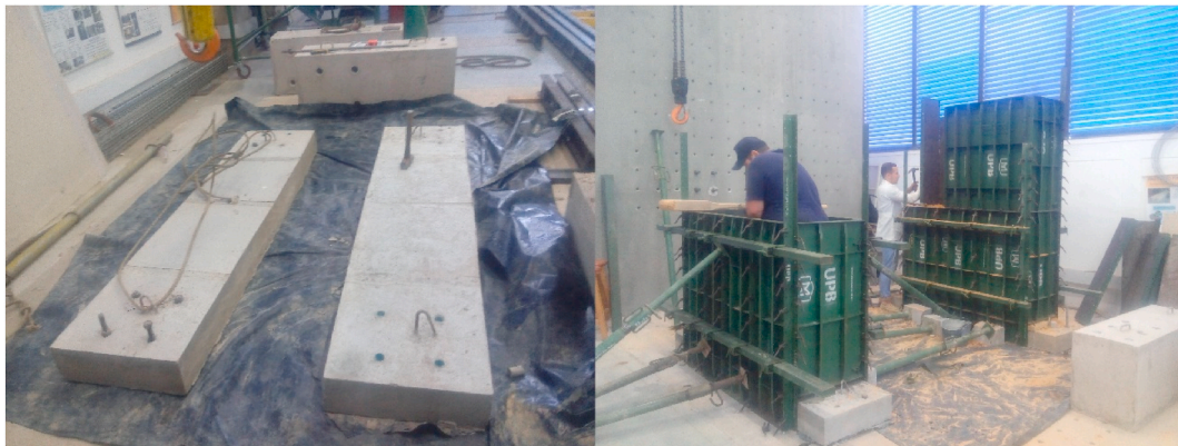
Fig. 2. Left: foundation and right: formwork.
