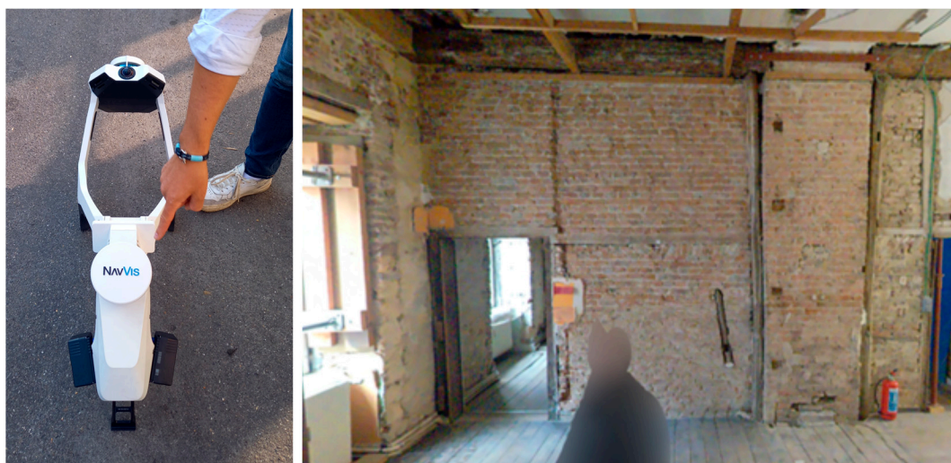
Figure 4. Case study 01: first-floor scan captured by the NavVis system, showing a half-timbered wall with brick infill. © Research lab Diva.
