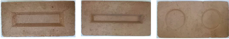
Fig. 1. Some examples of cavity-bricks found in Burkina Faso
