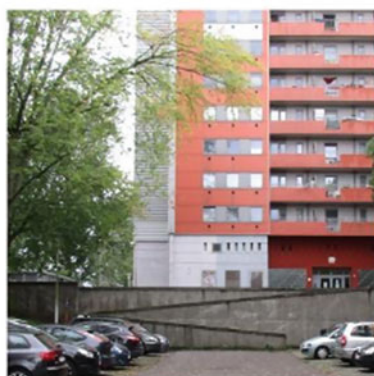
Stair and ramp system from the boulevard
