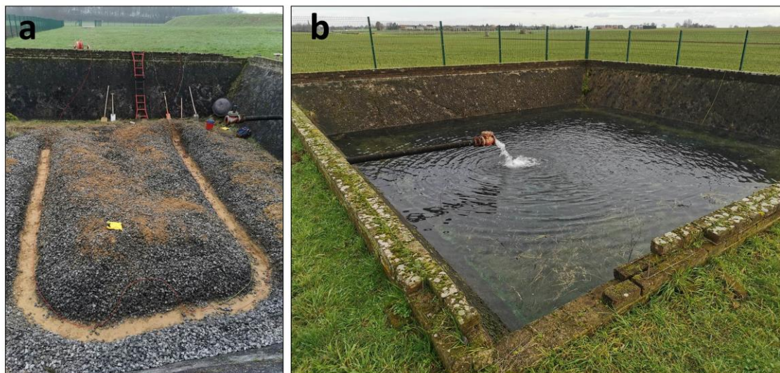
Figure 28. Infiltration basin during a) the installation of the FO cable and b) its replenishment.
