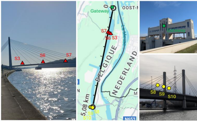
Fig. 7. The sensors fixed on the Lanaye Bridge and the Lixhe Bridge are respectively represented by red triangles and yellow circles. The gateway is placed inside a building and is represented by a green square.
