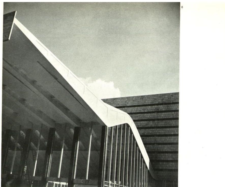
6, a detail of the reinforced-concrete roof of the booking hall which extends to form a canopy over the roadway in front of the station. Behind can be seen part of the office block. 7, general view of the booking hall and canopy. The curved shape of the beams follows the profile of the ruins of the Agger Serviano, as can be seen in 9, on the facing page.
