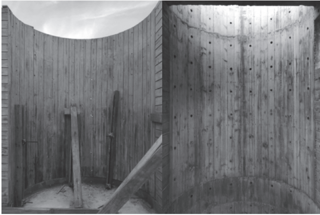
Figure 3. Pine Concrete House, ZA, Sugiberry ( Practices in Research , 1, front and back cover, 2020)
