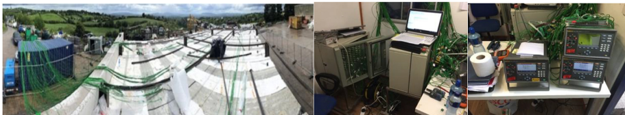
Plate 5. Extension cables for data sensors and data loggers
