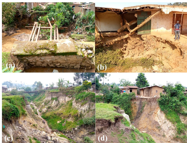
Fig. 6. Damages and economical losses caused by gully erosion expansion in the Kimemi watershed from (a) destruction of a bridge (b) commercial settlements, (c) gully expansion, and (d) poor households' vulnerability increase.
