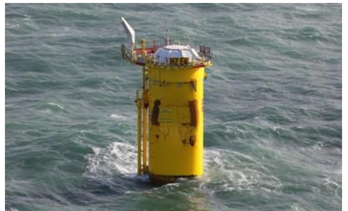
Figure 1. Damaged monopile foundation from the impact of a drifting cargo vessel (Dutch North Sea) - From (Hollandse Kust, 2022)
