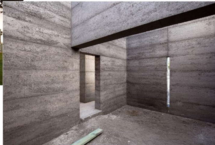
Rammed concrete for one-storey private house (Astbury, 2019)
