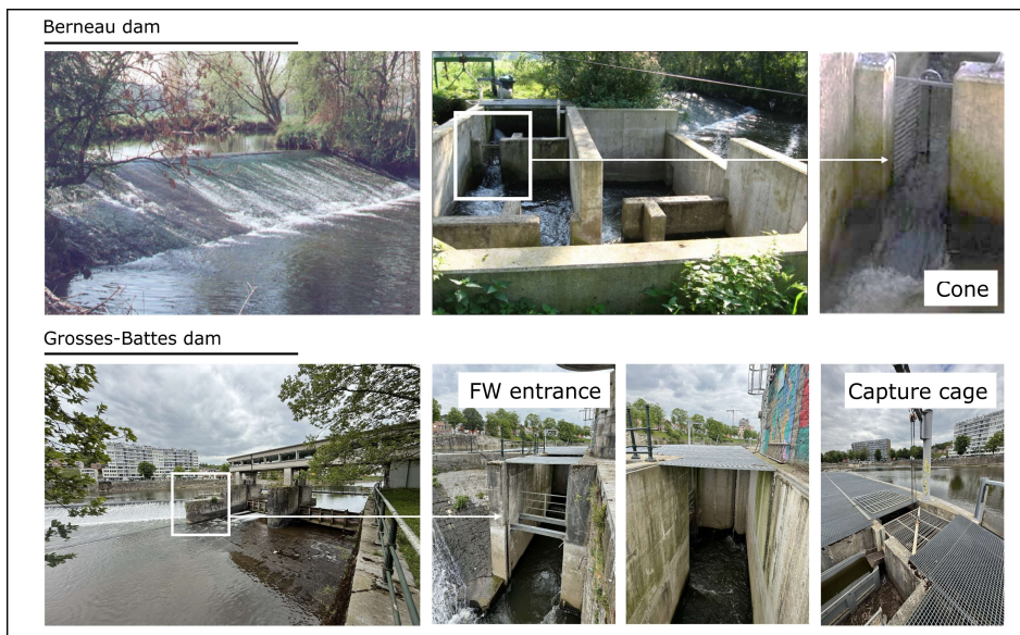
Figure 4. Berneau dam and Grosses-Battes dam site with the fishways and capture systems (basin with cone and cage).
