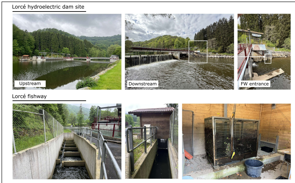
Figure 3. Lorcé hydroelectric dam site with upstream and downstream view of the dam, the fishway (FW) entrance and images showing the fishway and the capture cage.
