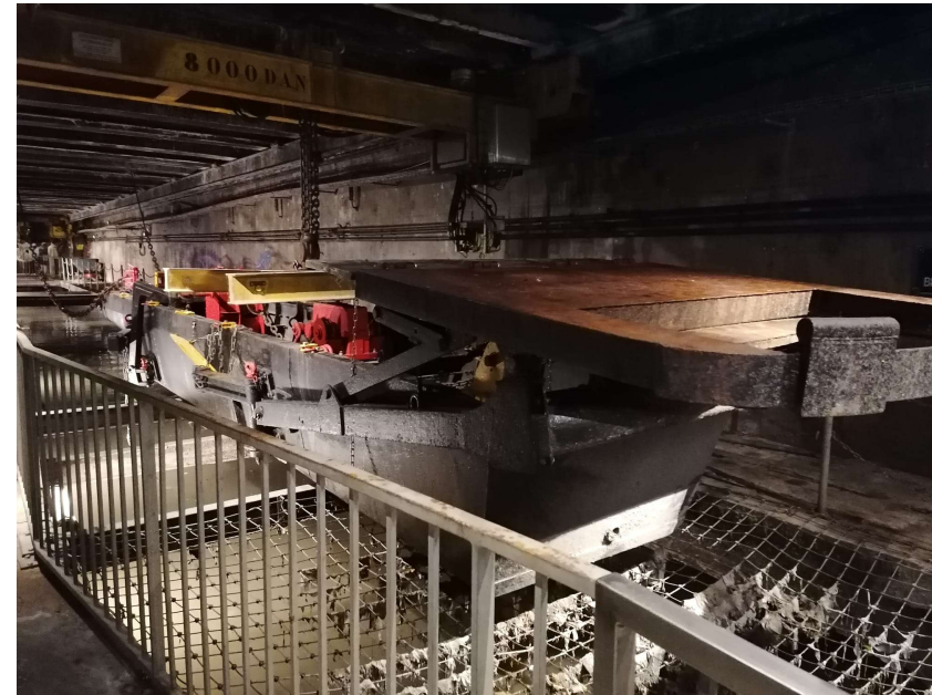
Paris sewers (France), with a sediment flushing boat
