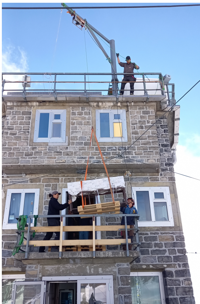
Figure 1: Removal on July 22, 2024, of the 120HR instrument via the balcony of the FTIR laboratory, using the hoist located on the upper Sphinx terrace. Picture E. Mahieu
