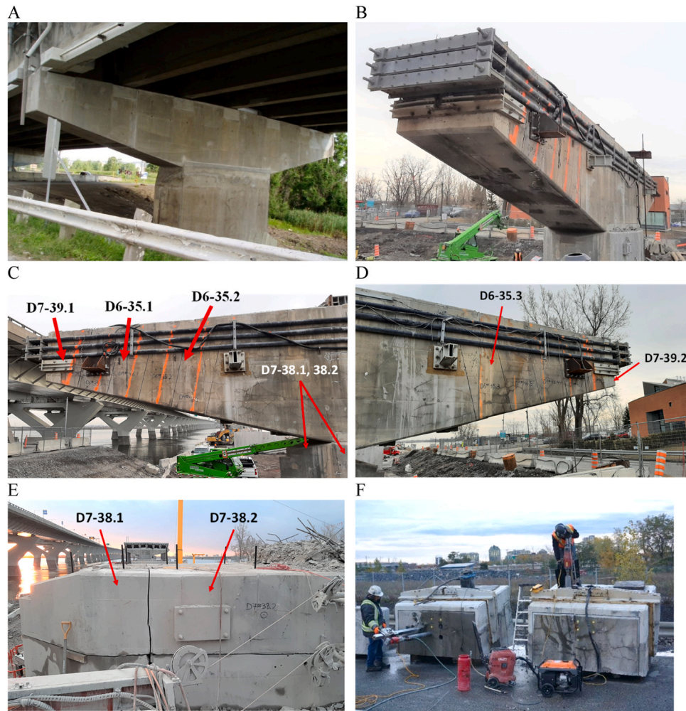
Fig. 2. Structural elements extracted from the Original Champlain Bridge and used in this study [photos from the study of Fournier et al. 2024 [46]]. A. Typical structural element on shore. B. Actual pier selected for coring showing external post-tensioning (repair conducted in 2008); the closest part of the pier cap corresponds to the North side of the structural element. C. Location of sections D7-39.1 (exposed) and D6-35.1 & 35.2 (protected under the bridge deck) in pier cap (North side); sections D7-38.1 and 38.2 in top of pier (north side). D. Location of sections D7-39.2 (exposed) and D6-35.3 (protected under the bridge deck) in pier cap (South side). E. Details of sections D7-38.1 and 38.2 in top of pier after complete removal of the pier cap. F. Coring of sections D7 39.1 (on the left) (exposed; North side) and 39.2 (on the right) (exposed; South side).
