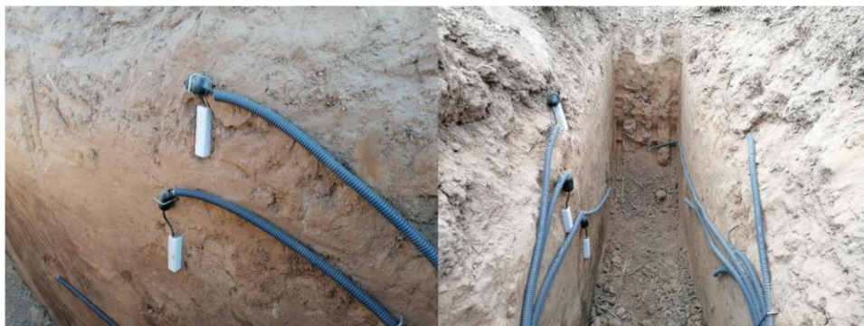
Figure 20. Protection and secure fixing of cables at the edges of trenches.
