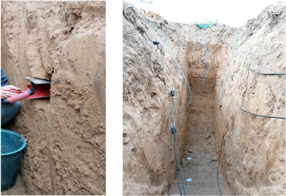
Figure 19. Installation of EcoTech soil water solution sampling plates at a depth of 1.2 m in the trenches of each plot.
