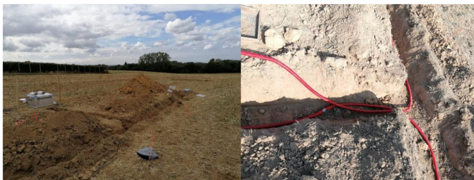
Figure 21. Illustration of the trenches allowing the cables from each plot to connect to the data loggers and the isothermal box located between two plots.
