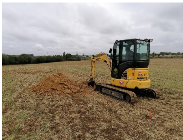
Figure 17. Excavation of 1.5-meter-deep trenches in each of the 8 plots.
