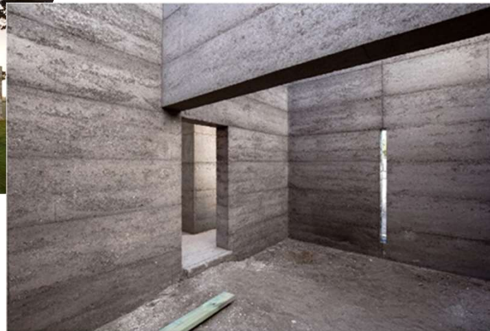
Rammed concrete for one-storey private house (Astbury, 2019)
