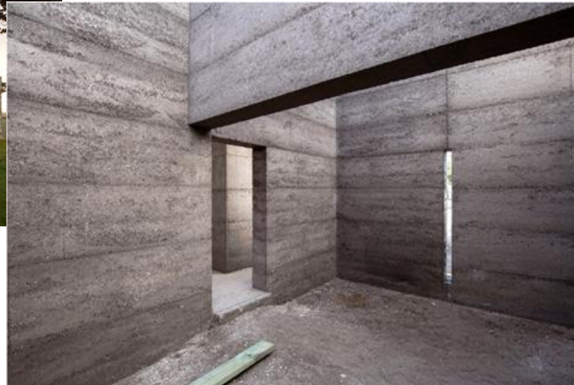
Rammed concrete for one-storey private house (Astbury, 2019)
