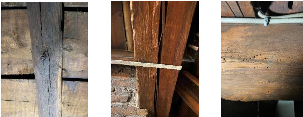
Figure 3. (a) Knots on a rafter from Place Emile Dupont. (b) Drying crack on a tie beam from Place Emile Dupont. (c) Wood-eating insect holes from Donceel hotel. Source: O. Noël
