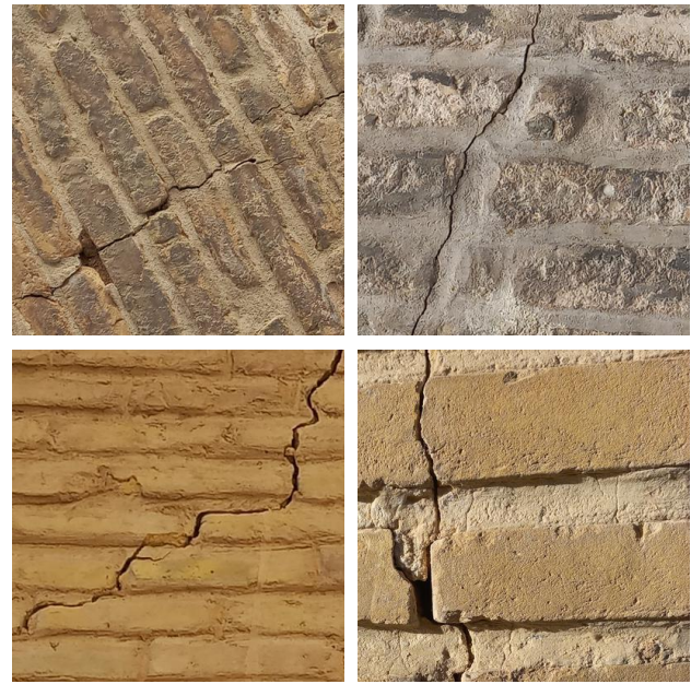
Figure 1. Example of masonry cracks used to train YOLOv5.
