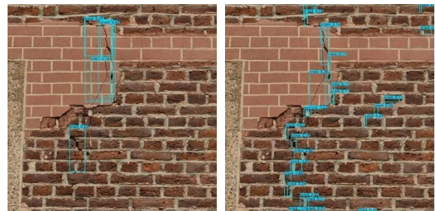
Figure 2. Impact of image resolution on predictions for the same crack
