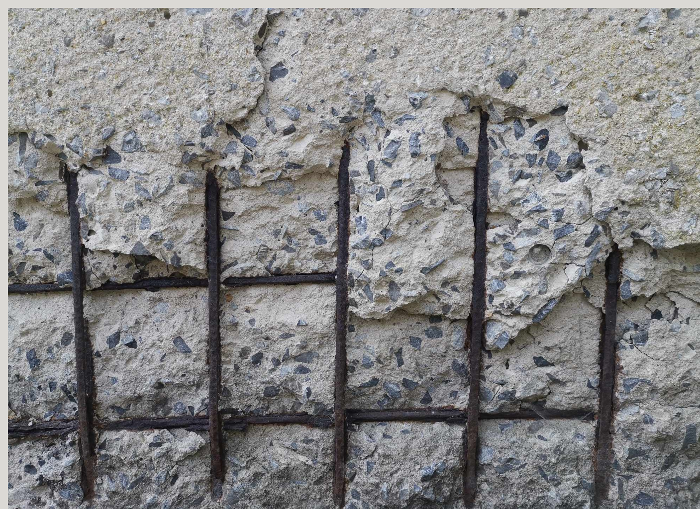
Figure 2: Corroded rebar in B6 Building (ULiège)
