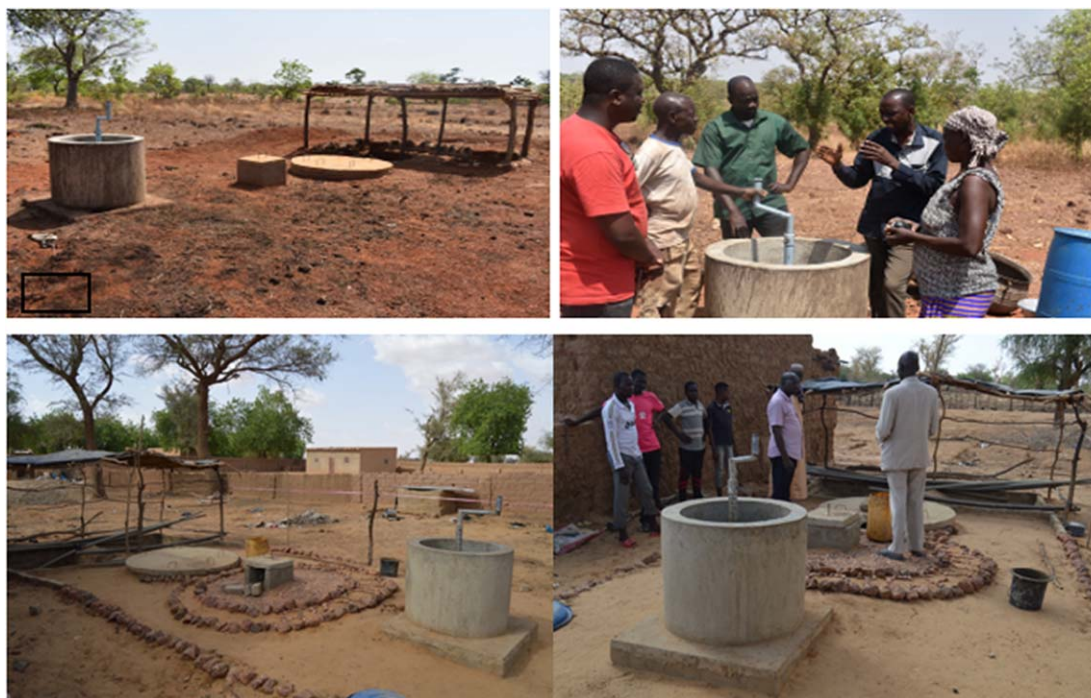
Figure 2. Completed construction of a biodigester (left) and a training session for recipients in Dano (Burkina Faso) and Bonkoukou (Niger) pilot sites. The slurry compost produced by the biodigester is used to support maize and millet production on the farm during all the rainy seasons.
