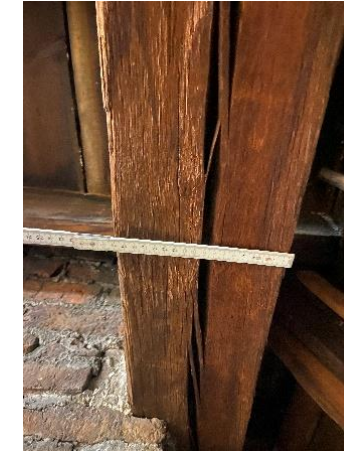
Source : Personal photographs of knots, drying crack and wood-eating insect holes of Donceel hotel and Place Emile Dupont, Liège.
