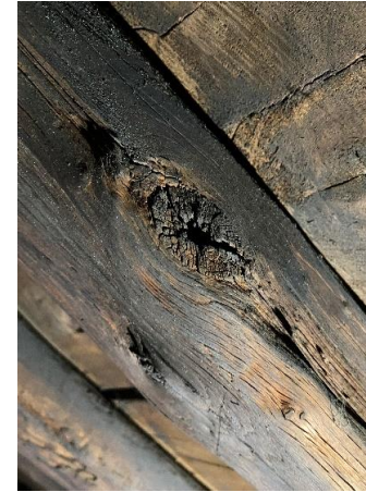
Source : Personal photographs of knots, drying crack and wood-eating insect holes of Donceel hotel and Place Emile Dupont, Liège.
