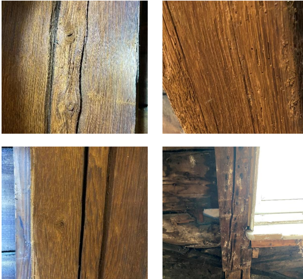
Source : Personal photographs of knots (1), drying crack (2 and 3) and wood-eating insect holes (4) of a Place Emile Dupont's rafter, Liège.
