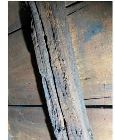
Source : Personal photographs of knots, drying crack and wood-eating insect holes of Donceel hotel and Place Emile Dupont, Liège.
