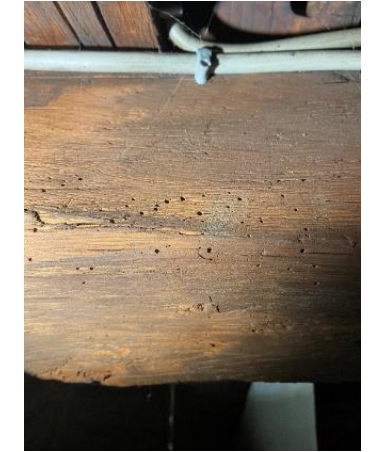
Source : Personal photographs of knots, drying crack and wood-eating insect holes of Donceel hotel and Place Emile Dupont, Liège.
