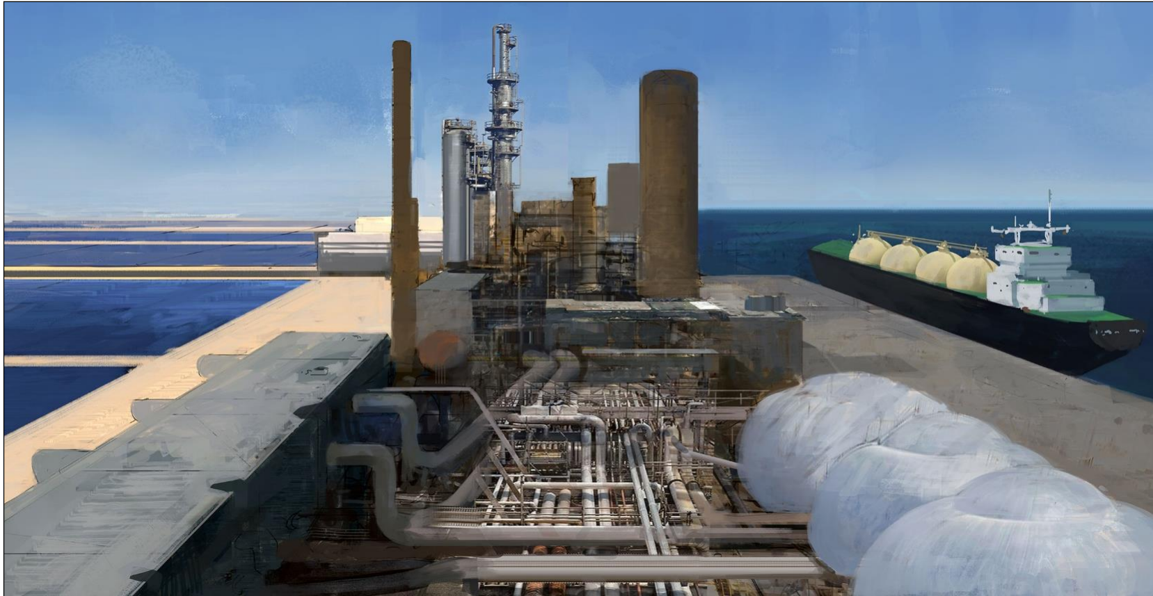
Artist's representation of an infrastructure where solar energy and direct air capture of CO 2 are used to produce CH 4 . The synthetic gas is then liquefied and shipped to consumption centres.
