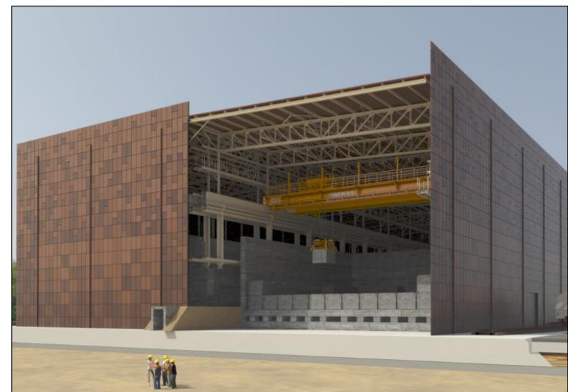
Concept of the future surface disposal facility in Dessel (Belgium) for LLW and ILW storage.
