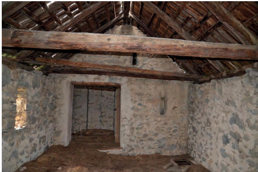
MR 1103, R+3, parement sud Cliché de V. Labbas, 2012
