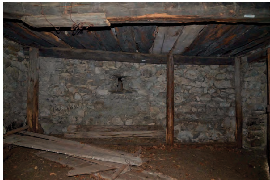
MR 1103, R+1, parement nord Cliché de V. Labbas, 2012
