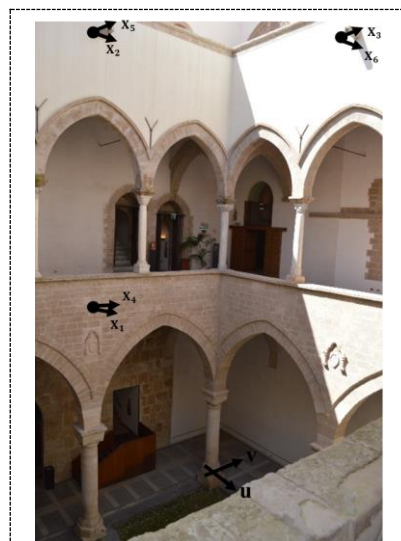
Figure 3. Position of the sensors
