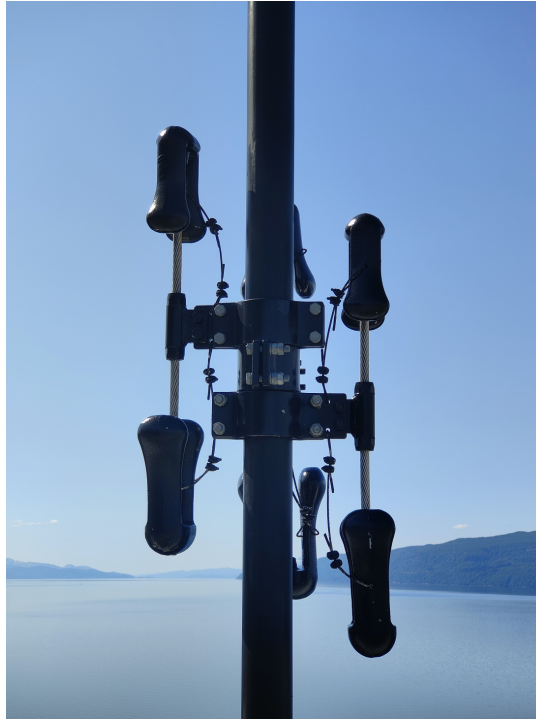
Figure 7: New configuration of dampers for the first three hangers from February 2022.
