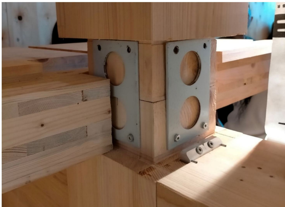
Fig. 1. Example of a bolted beam-column and slab-column connection that allows disassembling and reassembling.
