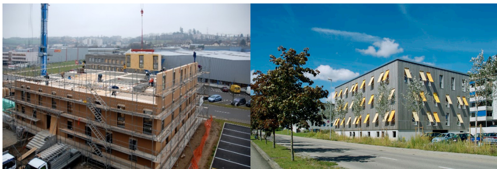
Figure 3.3. Second case study, the Green Office building [129]
