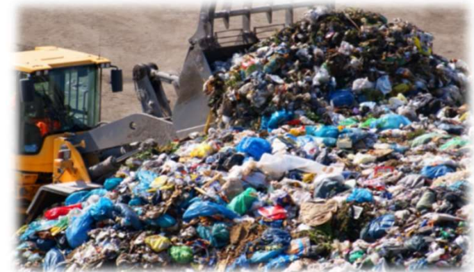
Piles of MSW
