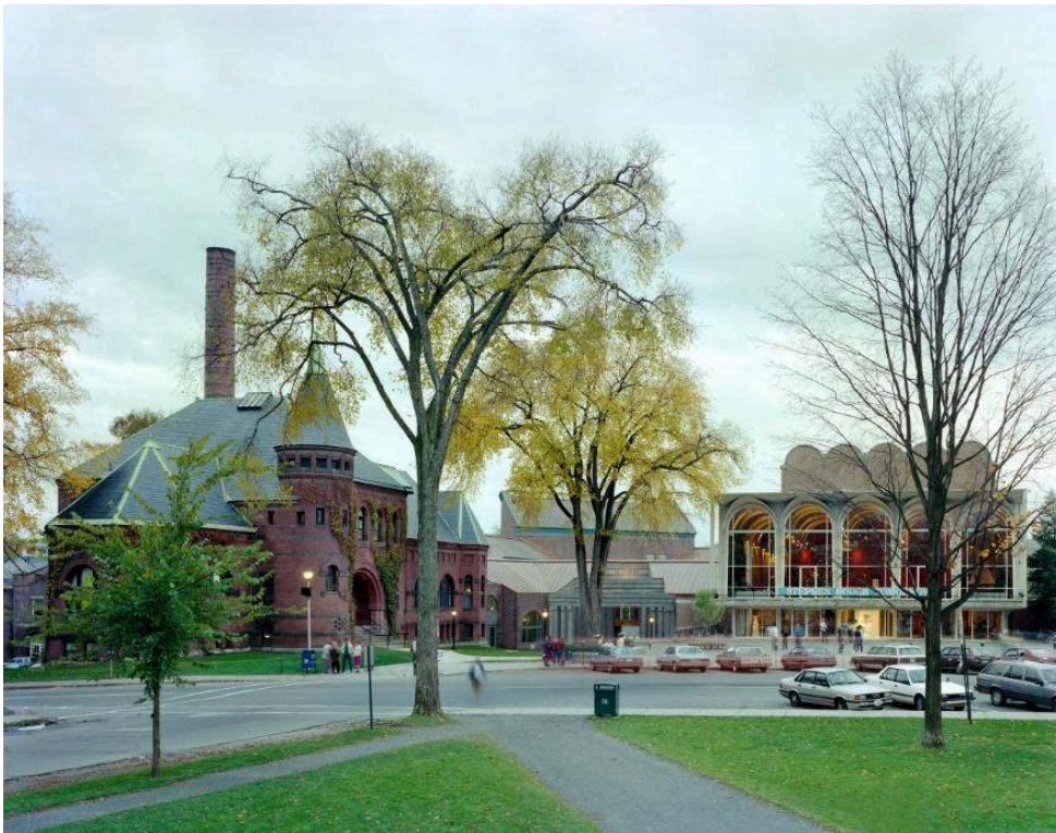
Charles Moore's original front facade of the Hood Museum in Dartmouth. From left to right: Wilson Hall, the Hood Museum and the Hopkins Centre.
