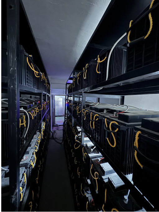
Fig. 7. ILMT UPS located in a room below the observatory floor.
