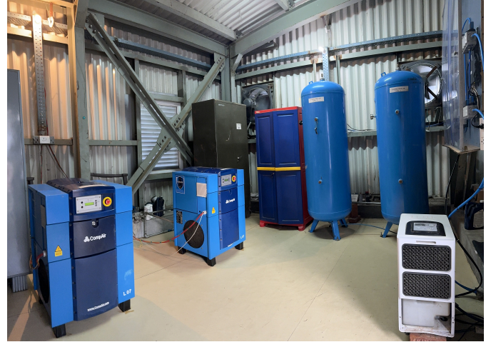
Fig. 5. Two independent and parallel air compressors and tanks are located in the compressor enclosure which is completely separate from the telescope building. Two exhaust fans are used to ventilate the room.
