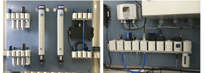
Fig. 6. Double air filtration systems located in the compressor room (left). A separate equipment combines air from each system, providing further filtration, pressure regulation and sensors (right). The latter equipment is located in the telescope control room.
