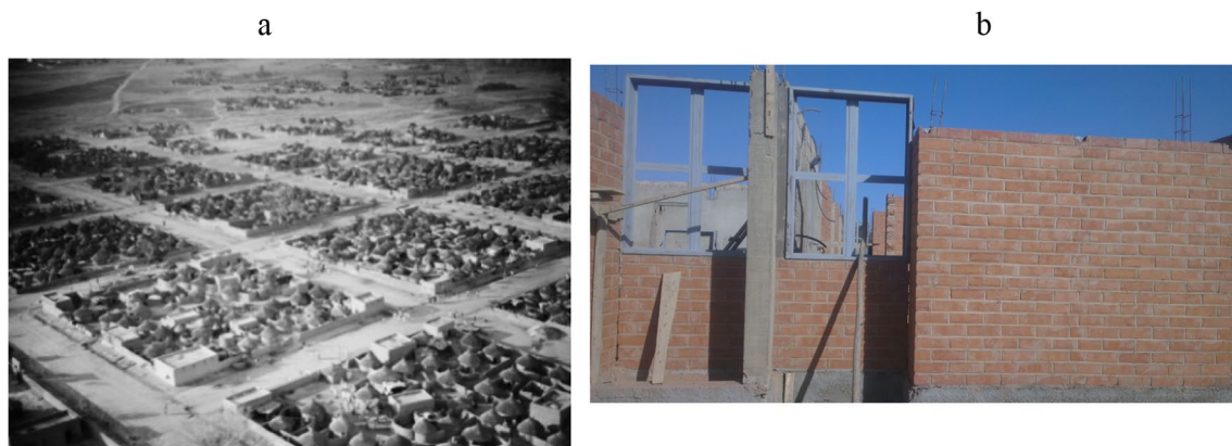
Fig. 1 Earth-based constructions in the city of Ouagadougou: a historical “Bancoville” in 1931; b contemporary construction using CEB in 2018 [3]
