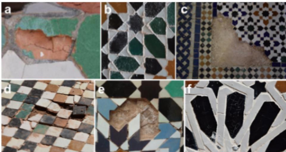
Time grains (a); soluble salts and cracks (b). Loss of tiles from the restored tiles at the Badi Palace (c, d, e). Restored zellige tiles from the Saadian Tombs revealing fouled cracks and uplifted pieces, causing surface irregularities (f).
