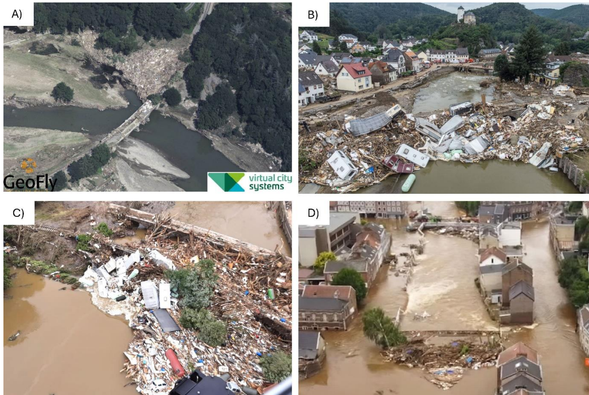
290 291 Figure 5 Examples of clogged bridges in the database. A) Pützfeld, Germany (bridge id 63 in the database, taken after the 292 flood). Photo based on an aerial survey by GeoFly GmbH and provided by Virtual City Systems. B) Kreuzberg, Germany (bridge 293 id 62, after the flood). Source: Baumert (2024). C) Altenahr, Germany (bridge id 55 and 56, after the flood). Photo by Polizei 294 Thüringen (2021). D) Pepinster, Belgium (foreground: bridge id 59; background: bridge id 60. During the flood) Credit: Vedia. 295 The flow direction is from left to right and foreground to background.
