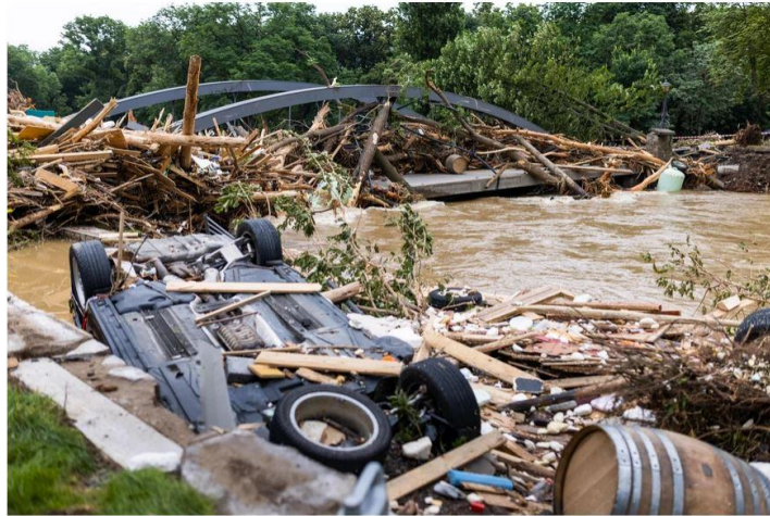
90 Figure 1: A debris accumulation in Bad Neuenahr, Germany (bridge 16 in the database by Epicum et al. (2024)). Trees, 91 vehicles, tanks and other objects are present in front and on top of the bridge, with debris interlocking with the bridge 92 superstructure. Photo by Philipp von Ditfurth (Jannaschk, 2021).
